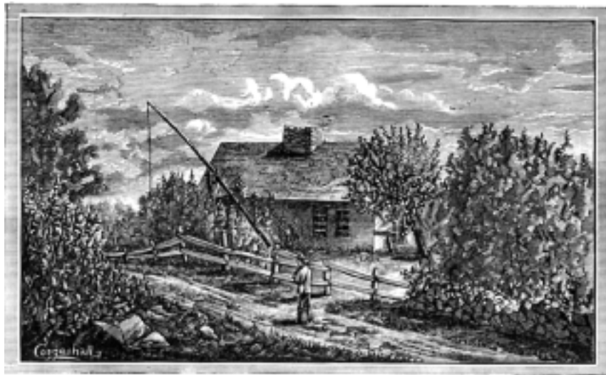
OLD BUTMAN HOUSE, BELVIDERE.
