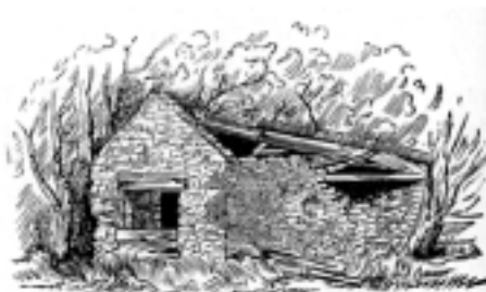
RUINS OF A CELLAR, BELVIDERE.
