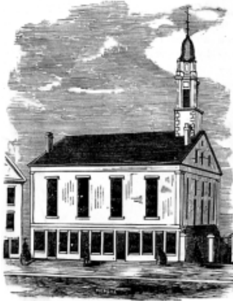
SUFFOLK-STREET ROMAN CATHOLIC CHURCH.
