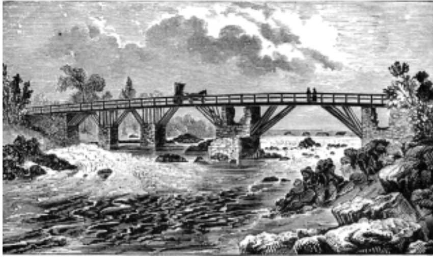
OLD BRIDGE OVER PAWTUCKET FALLS.
