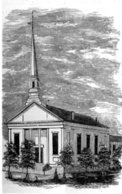
JOHN-STREET CONGREGATIONAL CHURCH.
