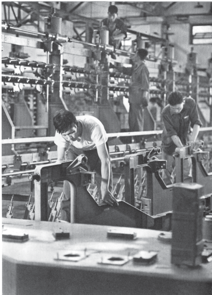
Installing a viscose filament spinning machine
