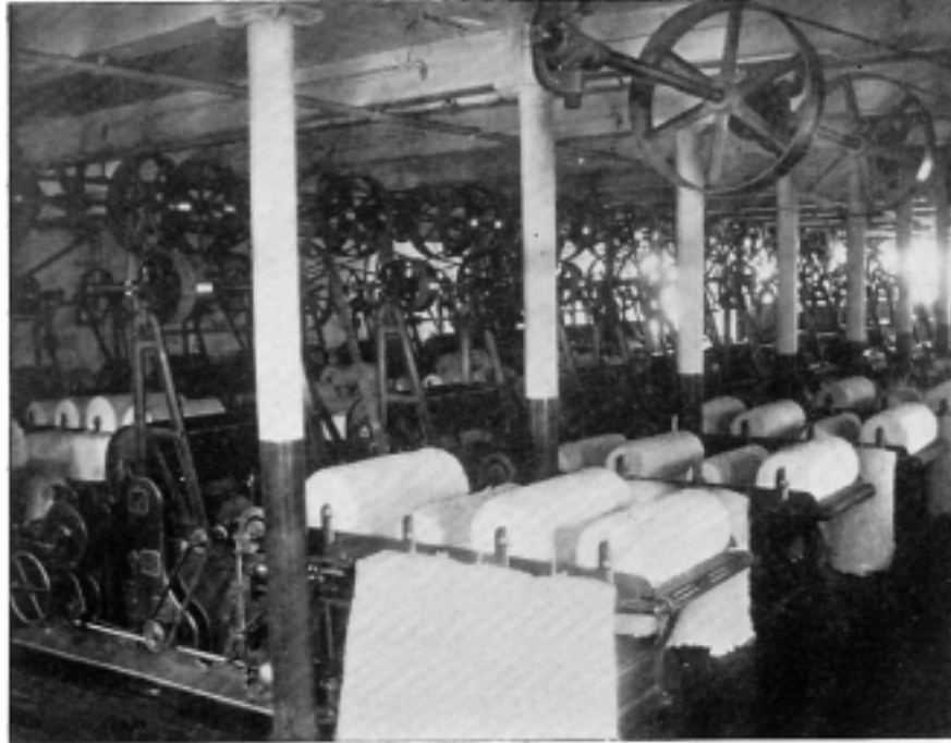
FIG. 11.—VIEW OF PICKER ROOM WITH BELT DRIVE, SHOWING MASS OF OVERHEAD WORK OBSTRUCTING LIGHT FROM WINDOWS
