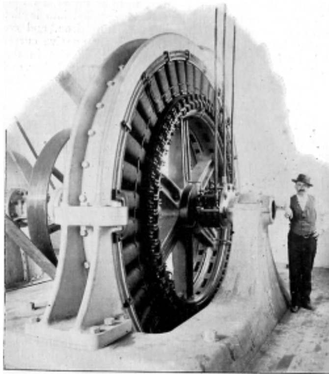
ANOTHER VIEW OF ONE OF THE BIG GENERATORS.
