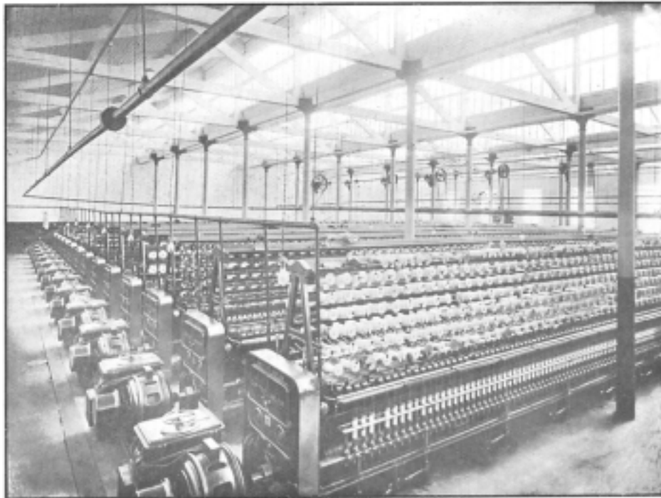
FIG. 9.—ELECTRICALLY-DRIVEN SPINNING FRAMES. DOBSON & BARLOW, LTD.
