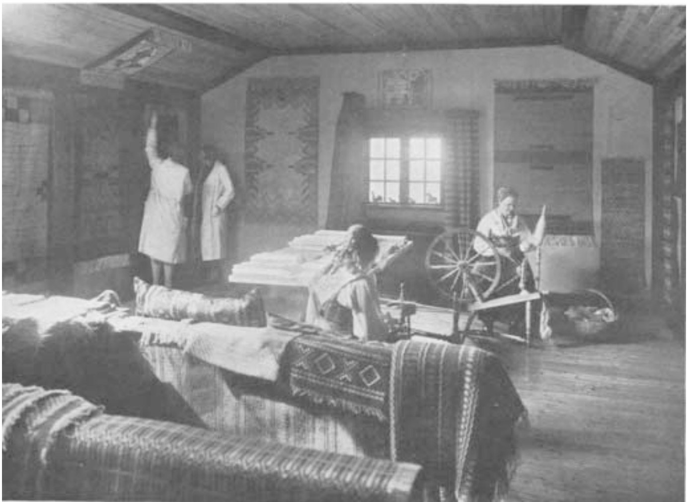
The showroom at the well-known Weaving-school, Sätergläntan
