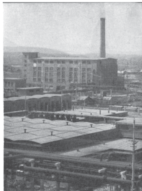
The Nanking Chemical Fibre Plant.
