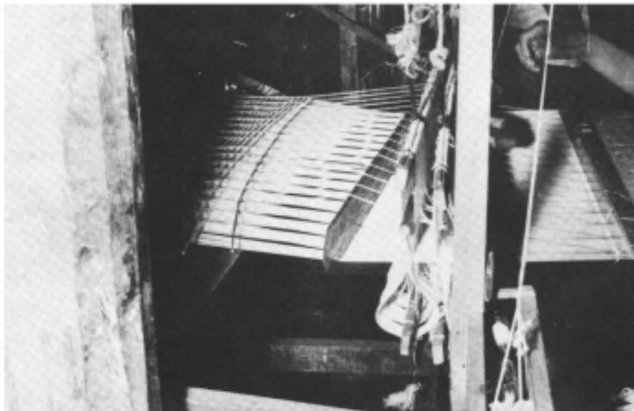
PLATE 3 — (Above) The “pattern-loom”. Lifting pattern-threads to form a warp-shed. Pattern-stick being inserted into the shed thus formed.
