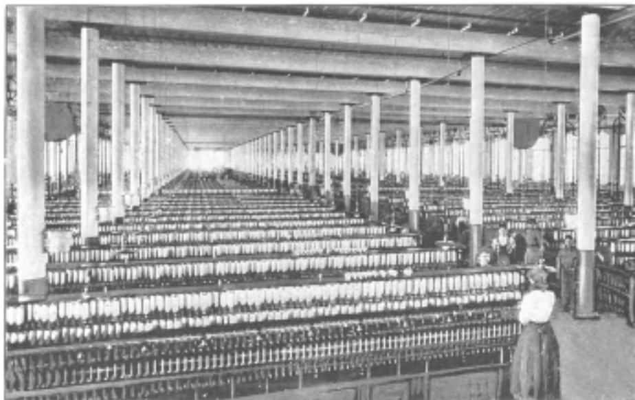
SPINNING-ROOM, SHOWING ROWS OF THROSTLES WITH SPINDLES AND FLYERS.
