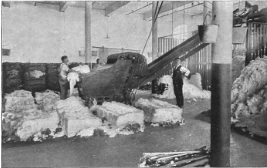
OPENING-MACHINE, OPENING RAW COTTON FROM THE BALE.
