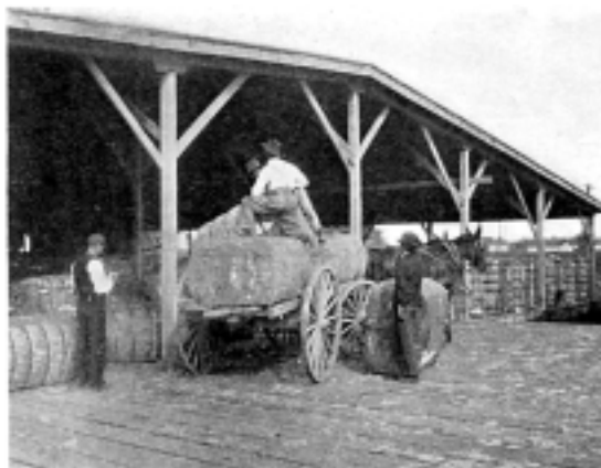
UNLOADING BALES AT THE COMPRESS
