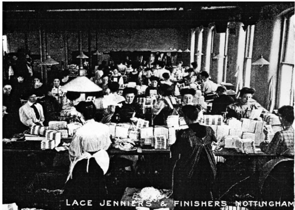
JENNIERS AND FINISHERS - These were at the tail end of the process, folding and putting finished lengths of lace onto card, with facings of coloured paper to set it off to best advantage in the haberdasher's window.
