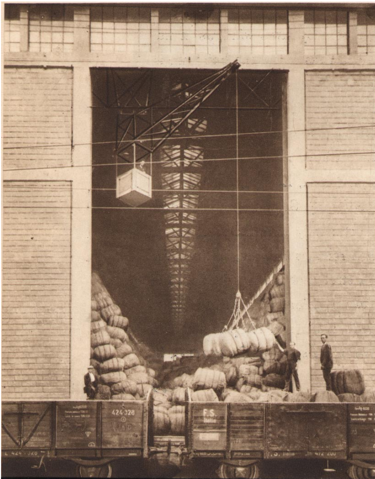
The Big Crane in the Warehouse
