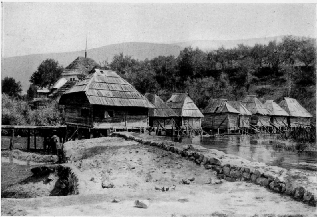
507 MILL HOUSES AT ILIDŽE
