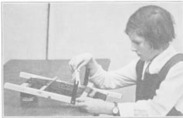
PLATE 15.—A FRAME LOOM FITTED WITH LEASHES.
