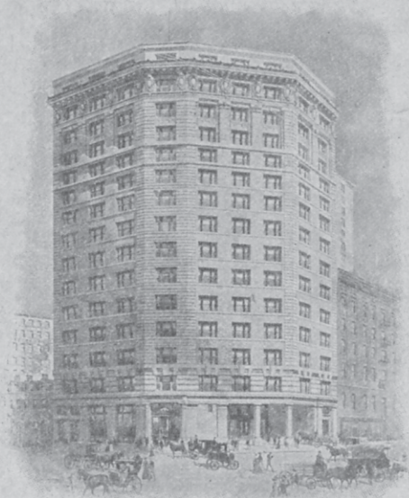
BUTTERICK BUILDING SPRING, VANDAM AND MACDOUGAL STREETS, NEW YORK
