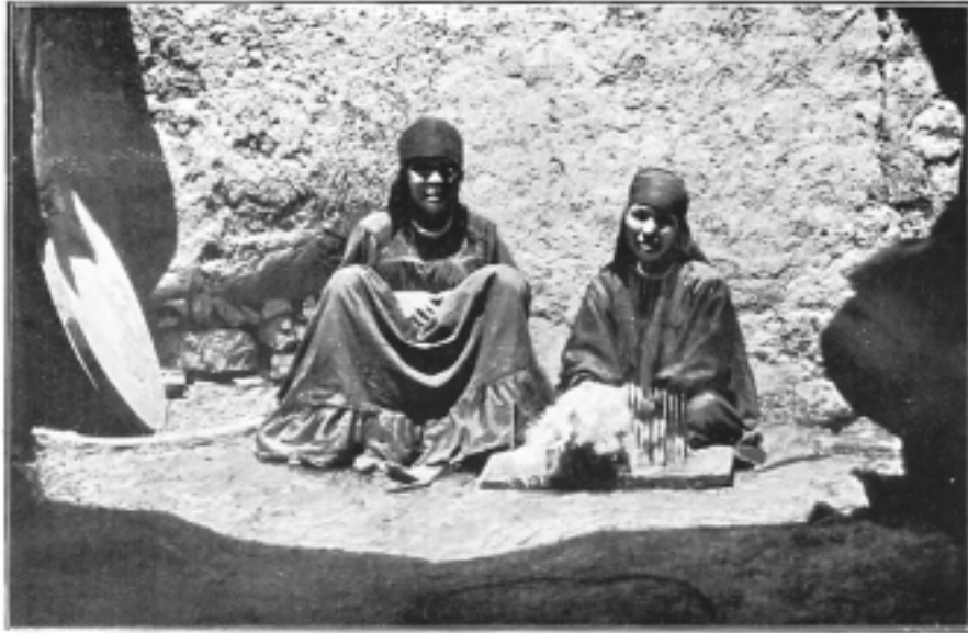
Plate 21.—HACKLING THE FLAX THROUGH A COMB WITH METAL TEETH.
