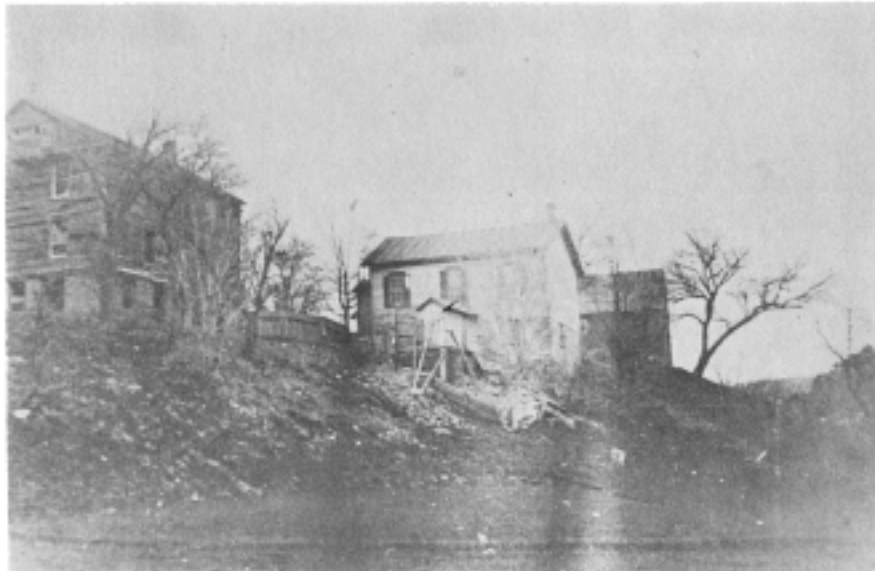
A rear view of the school – note the out house propped up with poles.
