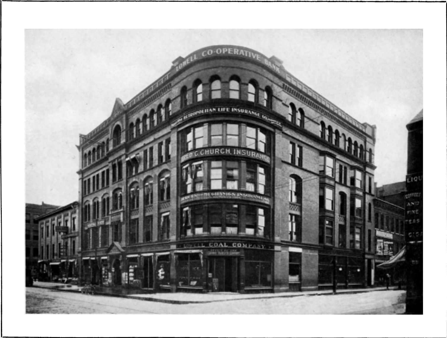
CENTRAL BLOCK, CENTRAL STREET One of the principal blocks, containing the offices of many of Lowell's professional men
